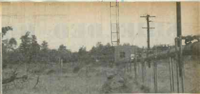
Power is fed to the tower through a feeder system extending several hundred feet to the transmitter house. The gin pole, hoisted together with its fastenings, to the top of the tower, is in two sections, assembled on the ground.
