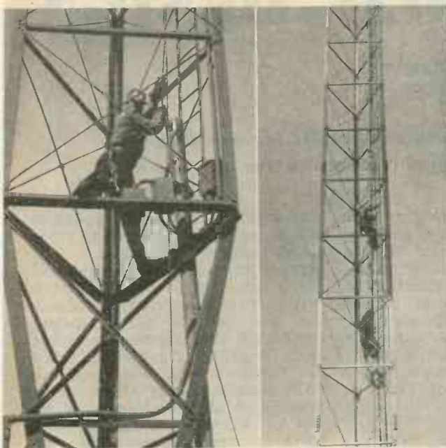
Gin pole is started up, remains inside tower
