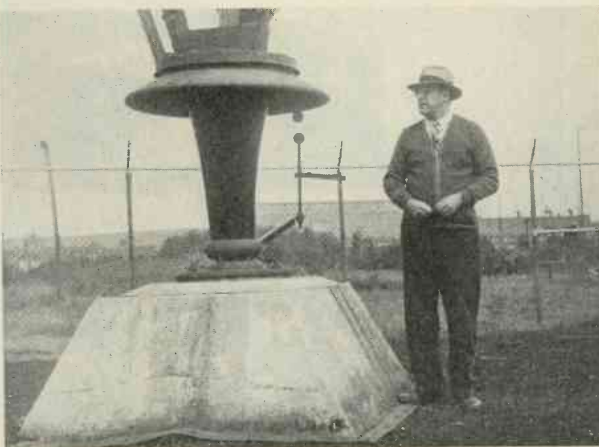
Approximately 150 tons pressure is supported by the base insulator, representing weight of tower and strain on guys; this bottom section is not dismantled but is merely unbolted from the foundation and transported to the new location.
