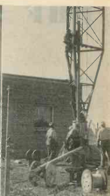
Raising first section of the 43 ft. gin pole
