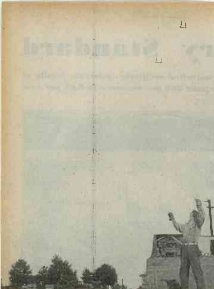
WJZ's guyed vertical radiator measures 640 ft.
